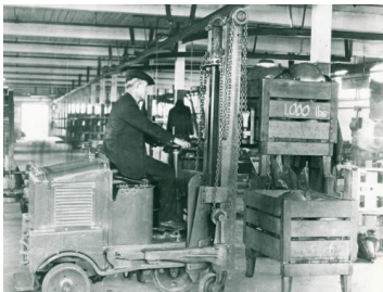
A modified Clark Duat - the first internal combustion forklift
